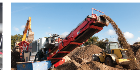
Extended main conveyor for massive stockpiling
