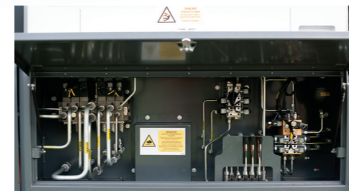
Steel pipework for better heat dissipation
