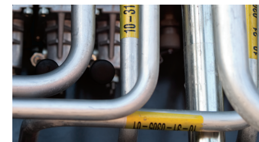
Steel pipework for better heat dissipation
